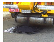
Laying asphalt mix
