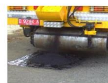
Laying asphalt mix
